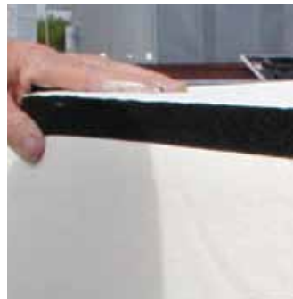
5. Apply ArmaTuff to top surface, overlapping the side pieces.
