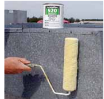
2. Apply thin, uniform coat of Armaflex 520 Adhesive.
