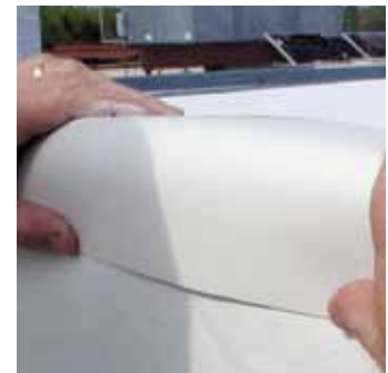
6. Seal and protect exposed edges and seams with ArmaTuff Seal Tape.
