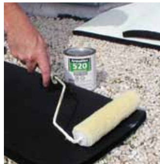
3. Roll thin coat of 520 Adhesive to insulation.
